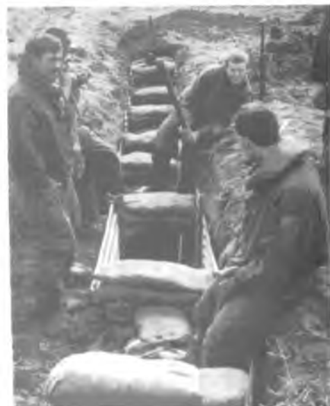
The split hairpin shelter, an eight man version off the vehicle and in the ground - Pie Stones (B Coy) waits for the platoon commander to come and tell him the trench is in the wrong position.
