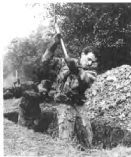
The split hairpin trench under construction.
